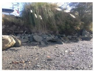
The seawall along Bay Road has some very old concrete plaster that is generally in good condition but there are several examples where remedial work is required.
