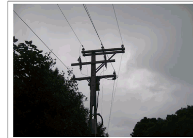
Vegetation near a pole in Excelsior Road
