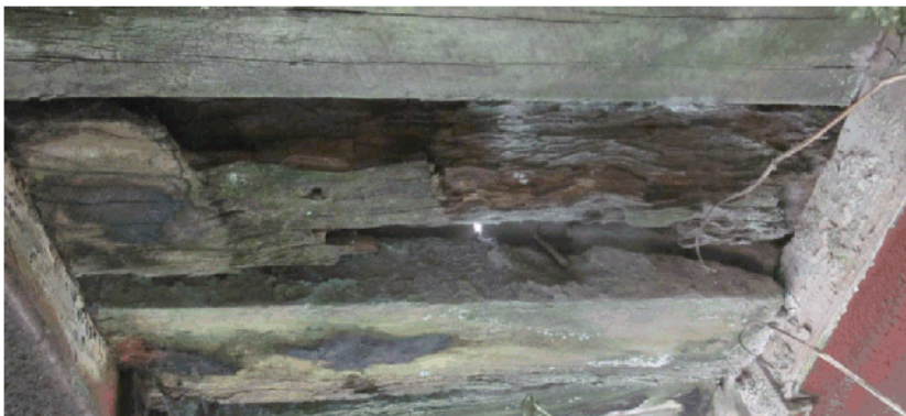
Photo showing state of some deck planks underneath bridge 1583.001.
