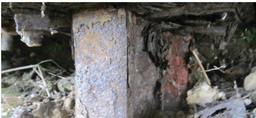
Photo showing rusty rail way iron piles support abutments underneath bridge 1583.001
