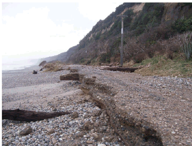
Figure 7-9: Coastal erosion of the Papatotara Coast Road along Te Waewae Bay (2007). Credit: Environment Southland.
