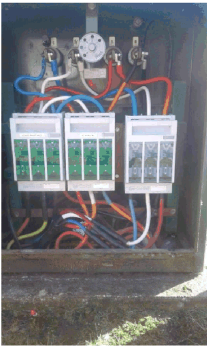
New transformer isolator (right side) for Heritage Centre connection
