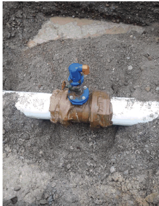
AIR VALVE FITTED TO KENT ROAD LINE
