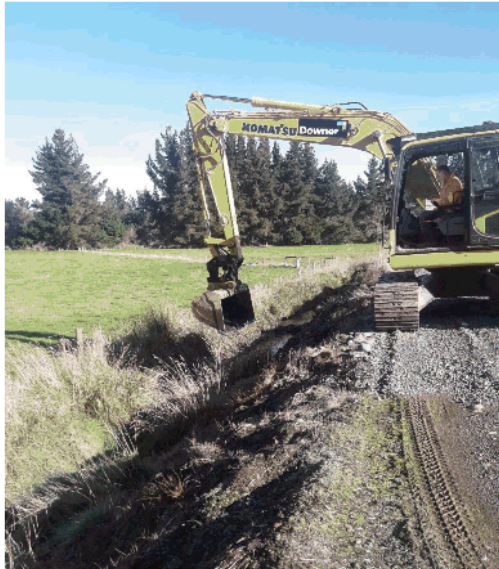
CLEARING OF DISCHARGE DRAIN FROM NIGHTCAPS PONDS
