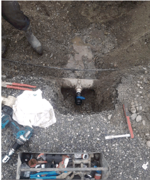
INSTALLATION OF 50MM OD RIDER MAIN 72 ROCKS HIGHWAY, RIVERTON
