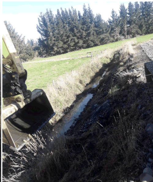
CLEARING OF DISCHARGE DRAIN FROM NIGHTCAPS PONDS
