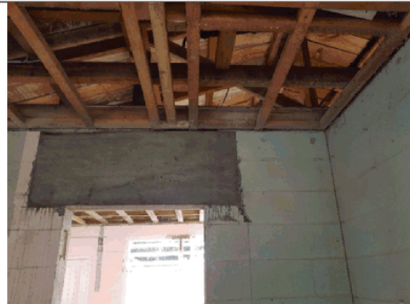
Photo 9: Lintel constructed during previous alteration
