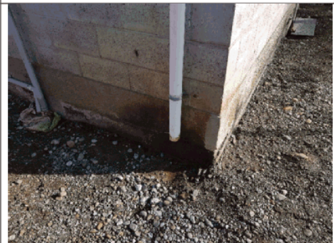
Photo 12 ; Stormwater dischsrgrin drivetly to ground.
