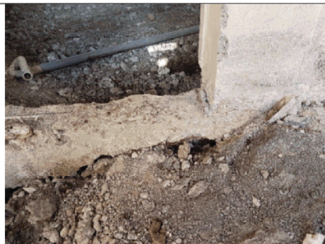
Photo 5: Void under footing, corroding reinforcing and spalling concrete.
