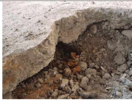
Photo 7: Voids under slab with timber present.
