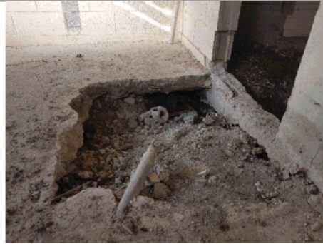
Photo 4: Voids under slab
