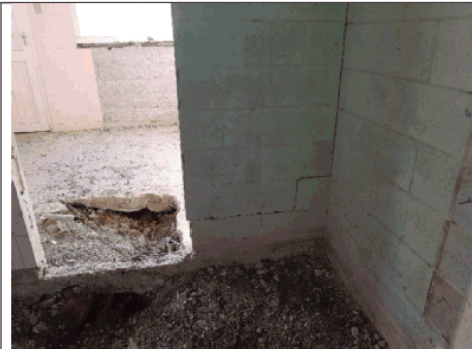
Photo 8: Movement in the jamb supporting lintel constructed during previous alteration. Evidence of unfilled blocks in jambs.
