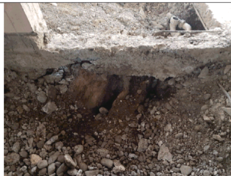
Photo 6: Timber present beneath footing.
