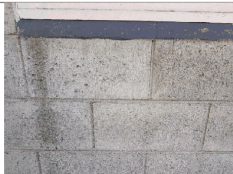
Photo 11: Staircase cracking in blockwork
