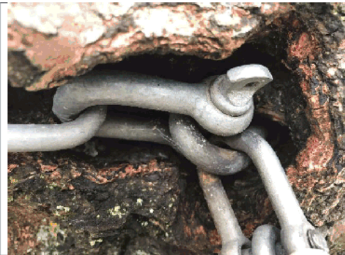
Tree growing over fixtures, can't inspect or replace them.
