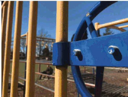
Bolt protrude at back of steering wheel
