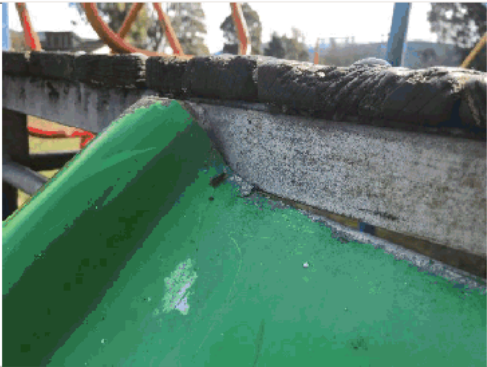
Gap at top of slide between deck – close this.
