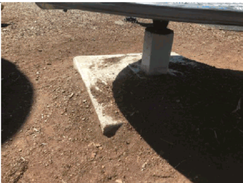
Exposed footing at slide runout
