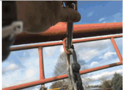
Finger entrapment in chain fixture
