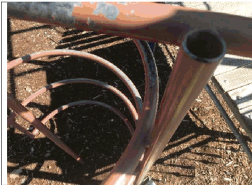
Pipe open on climber. Allows water to pool in footing and corode steel undetected.
