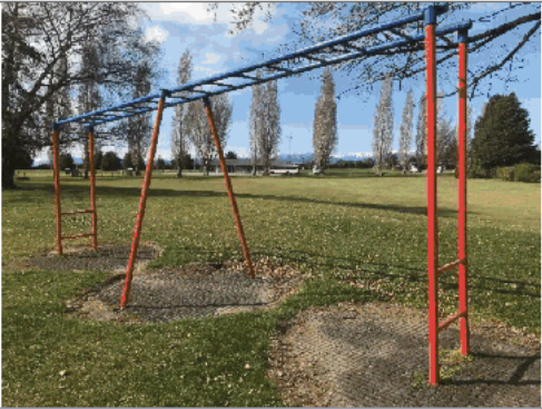
Overhead greater than 2.2high, inadequate impact surface
