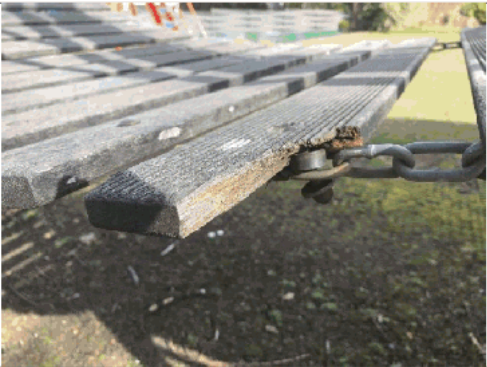
Timber broken on clatter bridge
