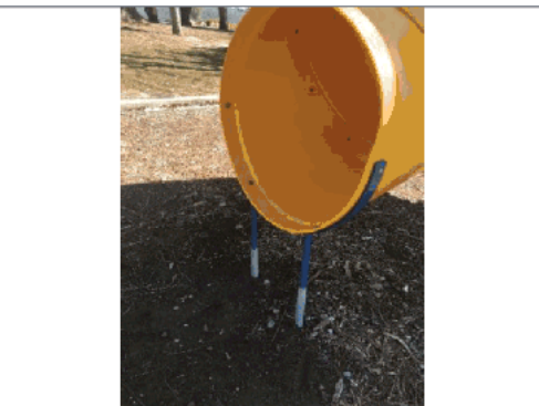
Tube slide has no runout
