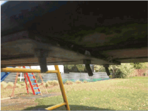
Protruding bolts under slide
