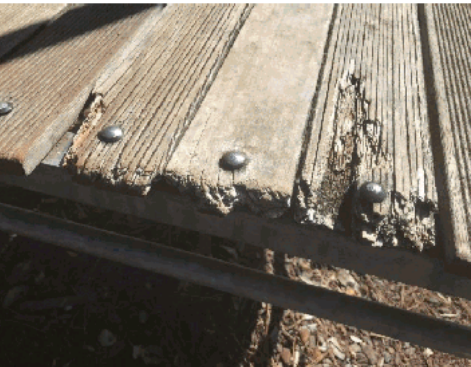
Deck rotting and broken
