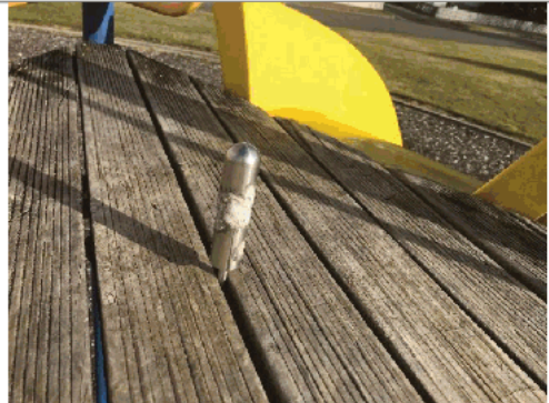
Finger entrapment in deck (forced movement at slide)
