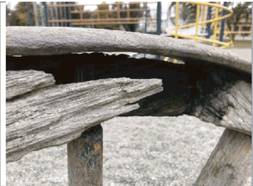
Wagon wheels on seesaw broken, sharp.
