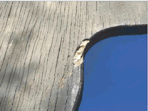
Plywood chipped
