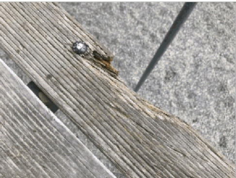
Deck broken and sharp
