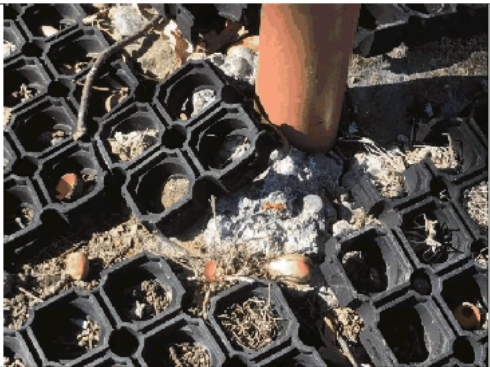
Exposed concrete footing
