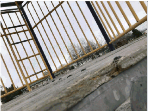
Deck broken in large high module
