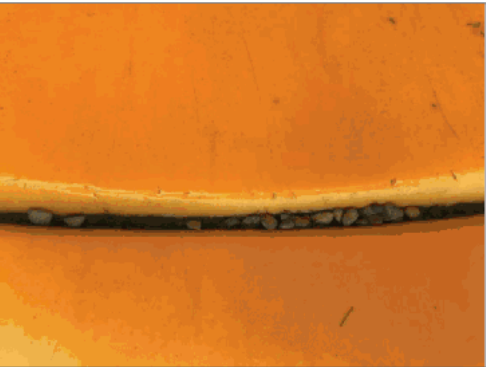
Peagavel stuck in slide joins
