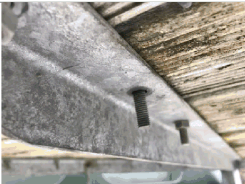
Bolts missing nuts and protruding
