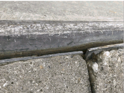
Skate plates at top of ramp bent out – can catch skateboard wheels
