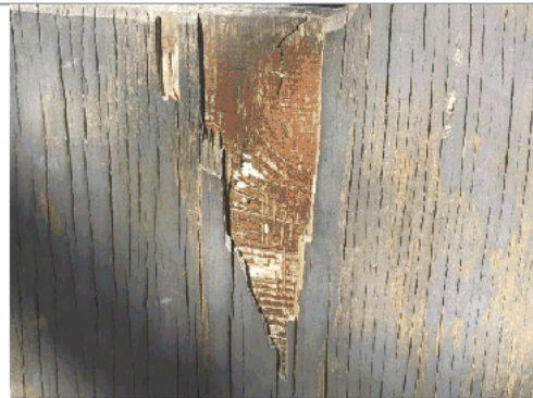
Plywood delaminating
