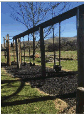
Inadequate surface for swings.
