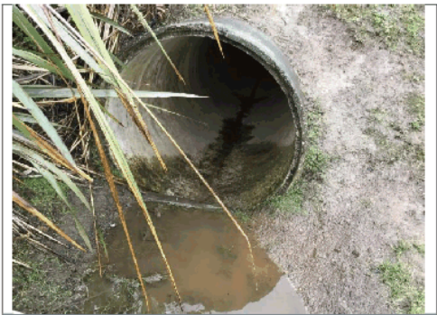
Water pooling at tunnel opening
