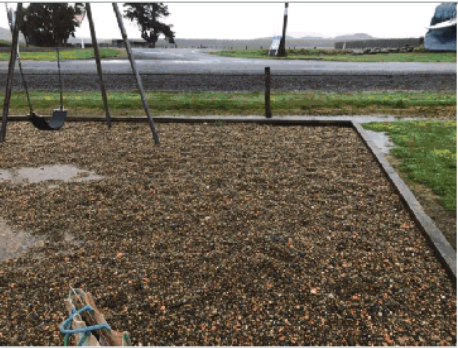
Insufficient fall space
