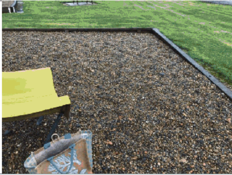
Insufficient fall space at end of slide.
