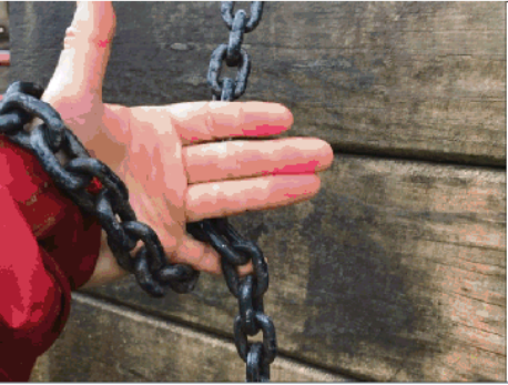
Chain on climber can be looped – entrapment
