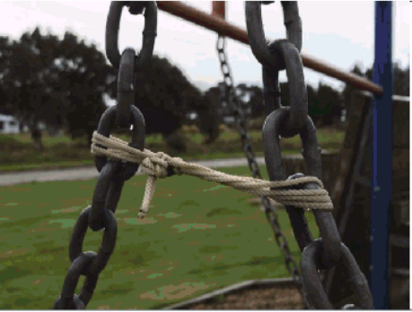
Remove string – creates and entrapment
