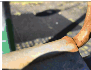
Swing plate lifting.
