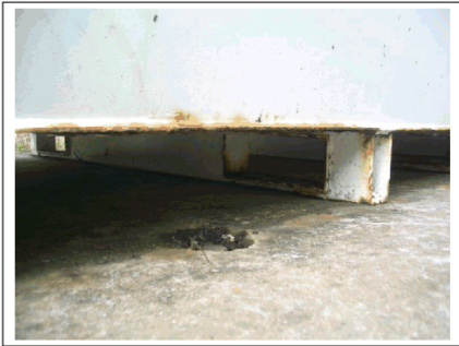
Rust on base of day fuel tank
