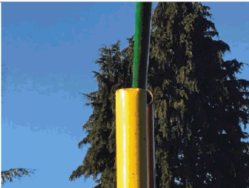
Pipe open – allows water to pool in footing and corrode undetected.
