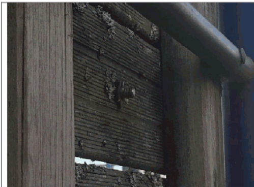
Protruding bolt on module
