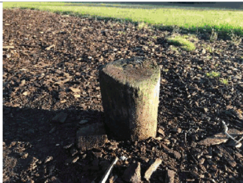
Seesaw buffer doesn't reduce impact in change of direction.
