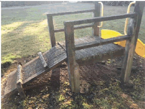
Easy accessible, deck over 600mm high, requires barriers (not guardrails).
