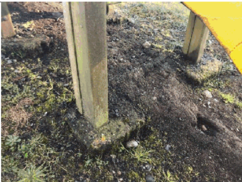
Exposed concrete footings
