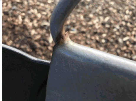
Swing plate burred and sharp
