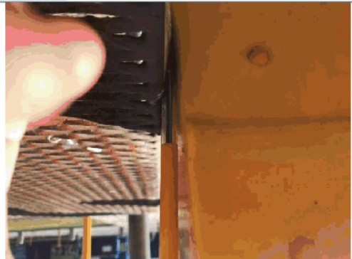
Toggle entrapment in gap between slide and deck
