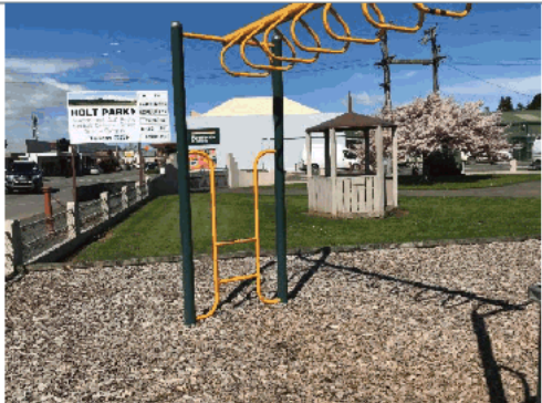
Ladder in fall space of overhead
