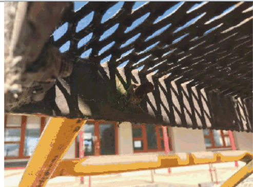
Protruding bolt under deck
