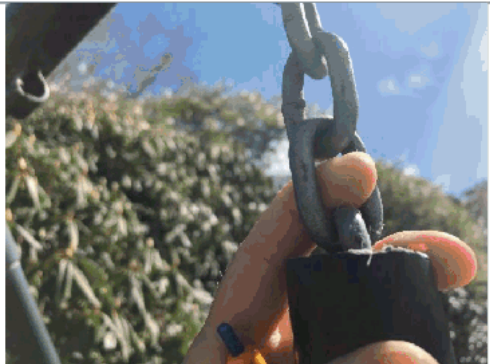
Finger entrapment in chains above hose
