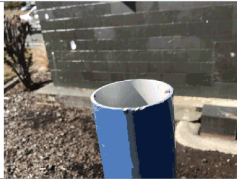
Pole open - allows water to pool underground in pipe and corrosion to go undetected.
