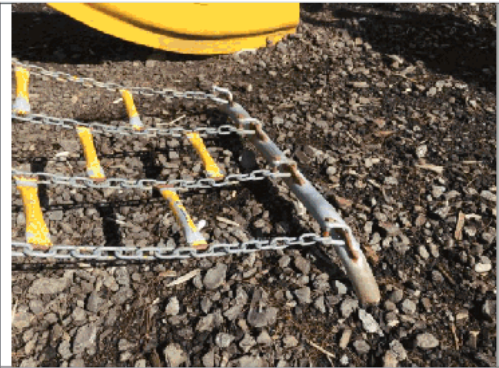
Solid object in fall space of cargo net
