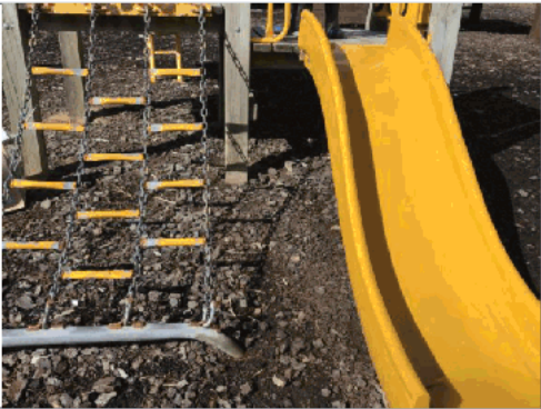
Cargo net too close to slide – in freespace and fall space.
