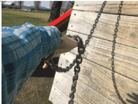
Chain nooseable on climbing wall
