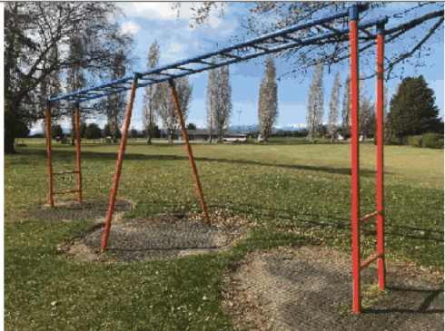
Overhead greater than 2.2high, inadequate impact surface
