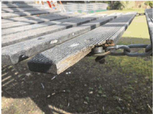
Timber broken on clatter bridge
