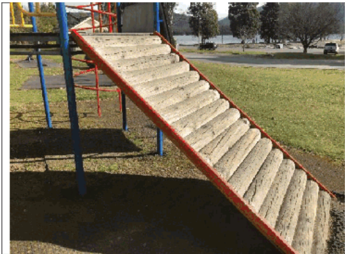
Steep play on easy accessible item requires opening no greater than 500mm
