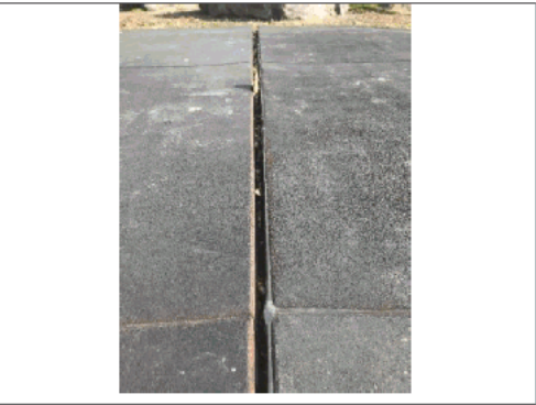
Gap in tiles – glue it shut.
