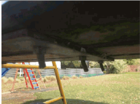
Protruding bolts under slide
