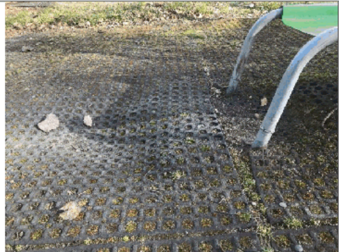
Runout surface VERY lumpy and hard.
