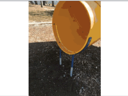
Tube slide has no runout
