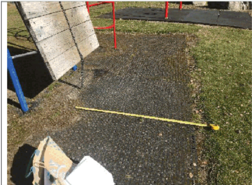
Insufficient fall space
