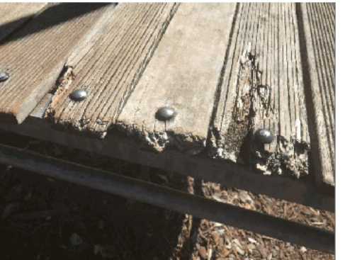
Deck rotting and broken
