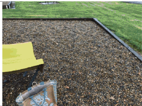
Insufficient fall space at end of slide.
