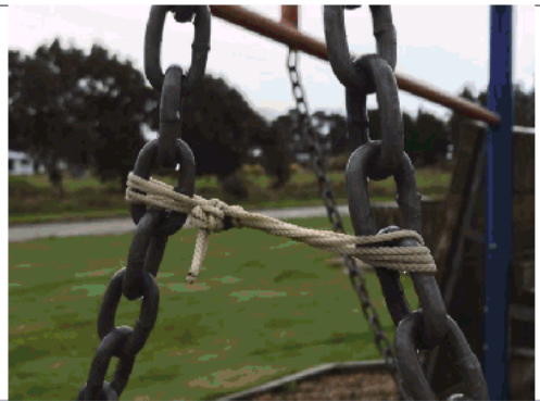
Remove string – creates and entrapment
