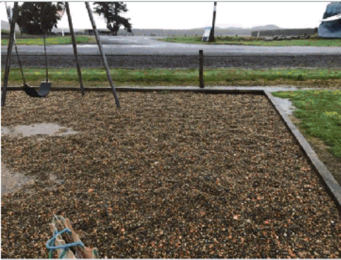
Insufficient fall space
