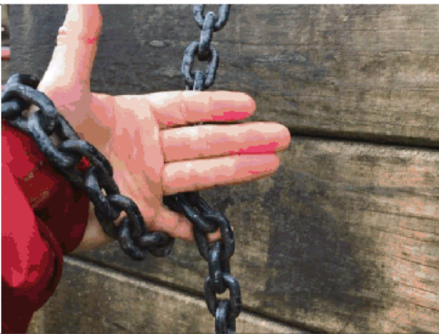
Chain on climber can be looped – entrapment
