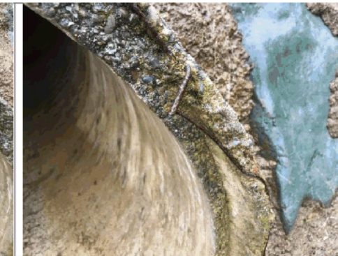
Wire exposed on tunnel opening
