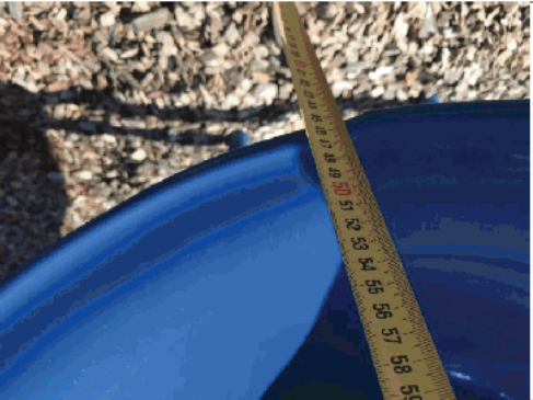
Run out of tube slide too high
