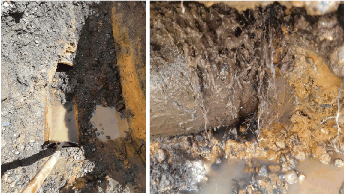
Church Street, Riverton – stormwater collapse and blockage
