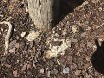
**Standard:** the depth of loose fill required is 200mm for a corresponding critical fall height of 2m. 300mm is required for a fall height of 3m.
