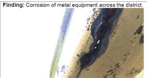
**Standard:** Metal parts should be protected against atmospheric conditions and cathodic corrosion.
