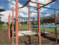
Standard: Falls over 600mm require impact attenuation in the fall zone.
