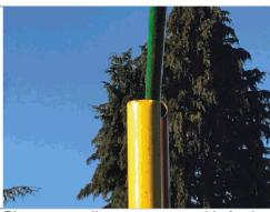
Pipe open - allows water to pool in footing and corrode undetected.
