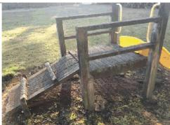
Easy accessible, deck over 600mm high, Evidence of deck measurement. requires barriers (not guardrails).
