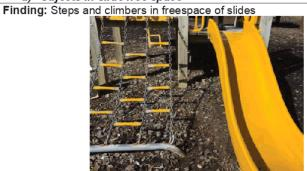
**Standard:** Free space in, on or around the equipment that can be occupied by a user undergoing a movement forced by the equipment (e.g. sliding, swinging, rocking). Climber fall space shall not overlap freespace.
