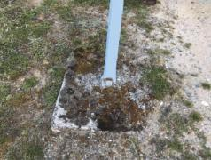
Exposed footings, swing frame appears damaged/bent.
