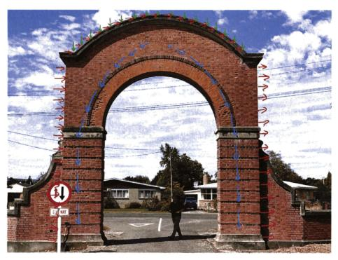
Figure 4: Typical Lateral Load Path Diagram in the E-W Direction.
