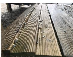
Deck warped and raised.
