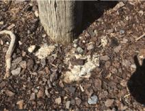
**Standard:** the depth of loose fill required is 200mm for a corresponding critical fall height of 2m. 300mm is required for a fall height of 3m.
