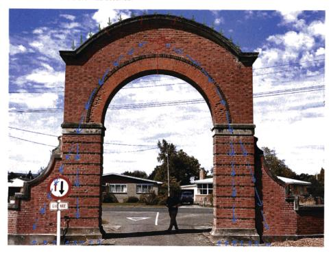
Figure 1: Typical Gravity Load Path Diagram for Archway (Cracking shown in red)
