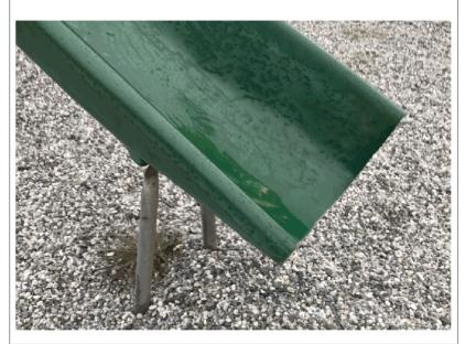
Standard: All slides shall include a run-out section.
