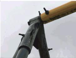
Protruding bolts on swing – cut down and cover
