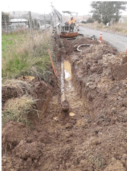
Mains burst repair Nightcaps
