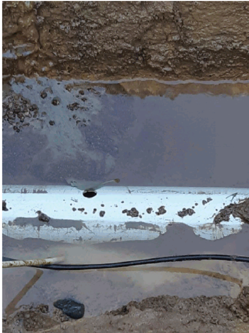
Hamlet Street, Riverton – illegal penetration into sewer network
