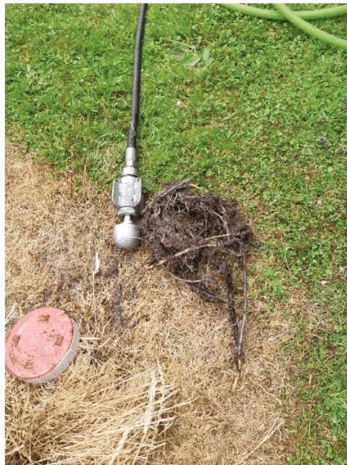
Tree roots removed from lateral junction to the main at Ohai
