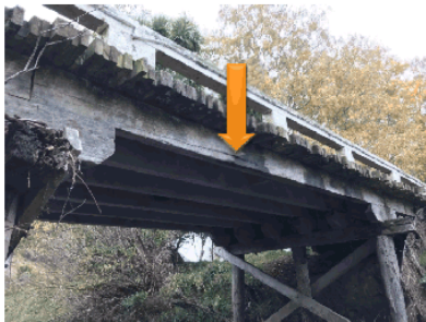
Figure 4-5: Cavity with splitting in D/S beam
