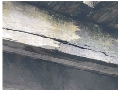
Figure 4-6: Close up of the cavity hole with splitting extending along the beam.
