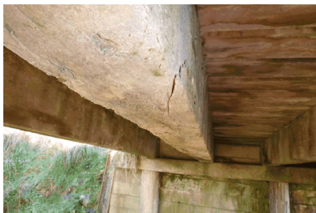
Figure 4-9: Split on beam 4 of Bridge 1253.001 Badwit Rd. Ongoing monitoring is required.
