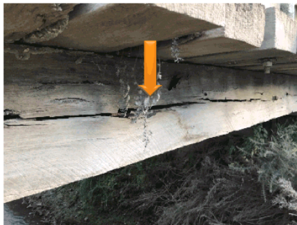
Figure 4-7: Existing splitting in D/S beam
