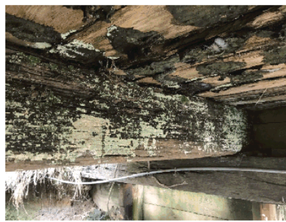
Figure 4-2: General decay and fungal attack of beams
