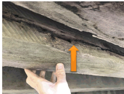
Figure 4-8: Close up of the replacement beam adjacent to original.
