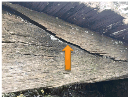
Figure 4-3: Shear split of U/S beam on outside edge
