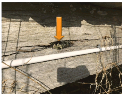
Figure 4-1: Cavity with splitting in D/S beam
