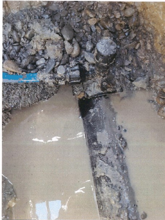
150 PE saddle failure – 31 Prince Street, Winton
