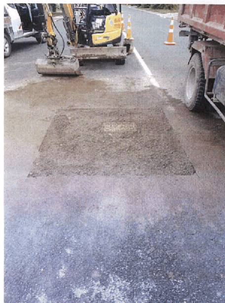
Fire Hydrant Replacement Matai Street, Te Anau
