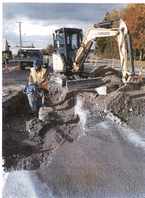
300mm valve replacement on Milford Road
