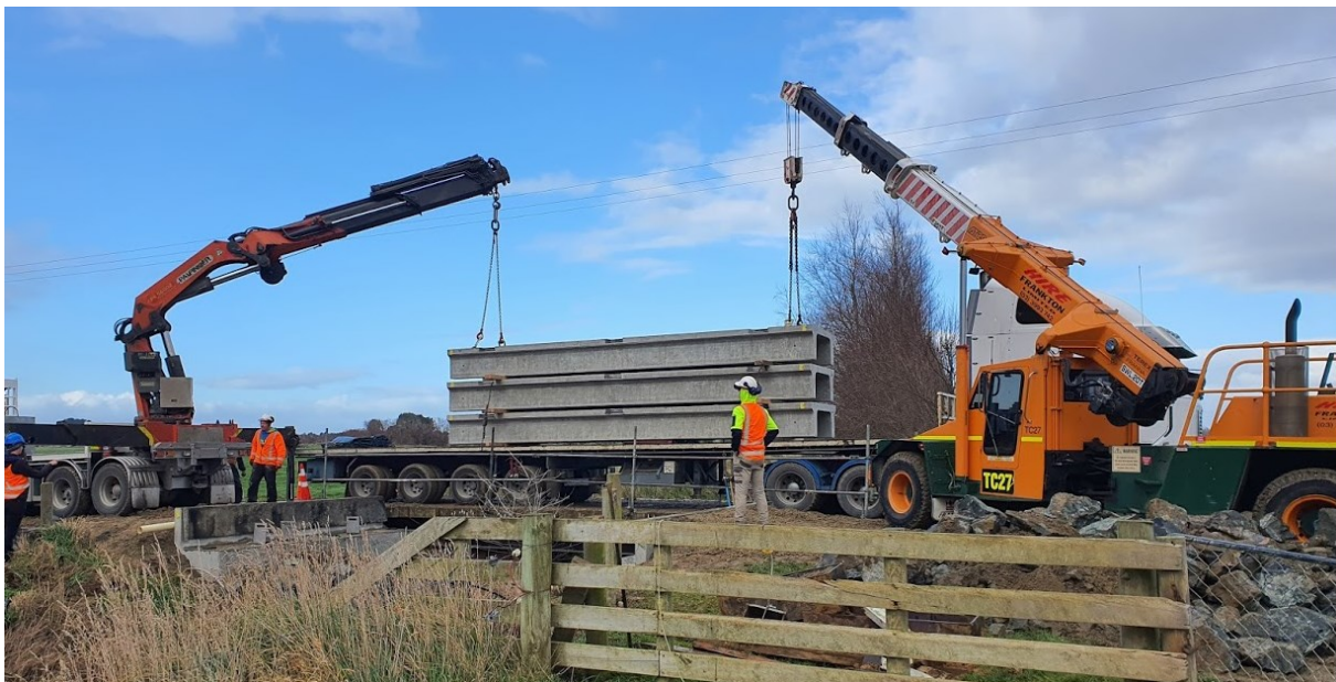
Installing beams at Pullar Road
