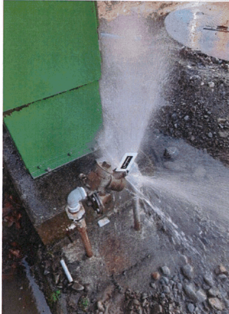
BFP Leak in Otautau
