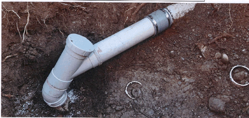
Foul sewer repair Mokonui Street, Te Anau
