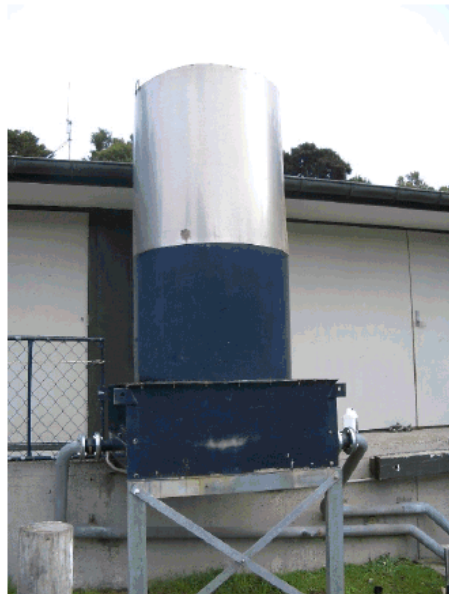
Unit two radiator relocated to serve Unit 1
