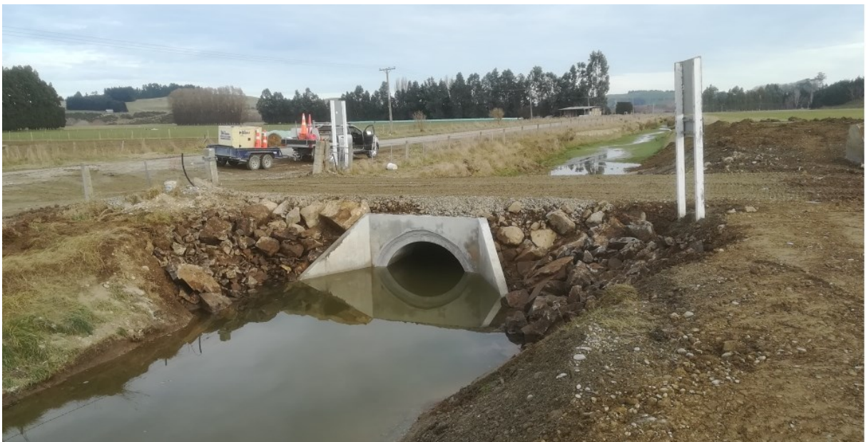
Culverts at Ardlussa Cattleflat Road under construction
