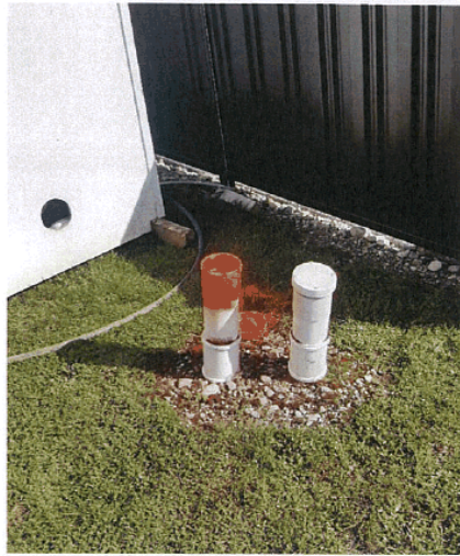
Sewer/stormwater identification on new building site
