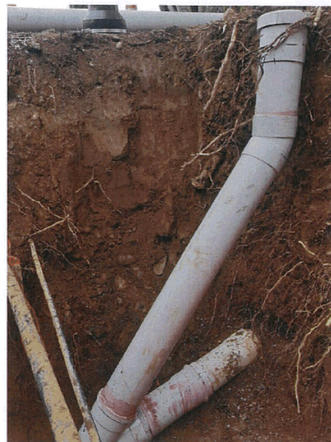
Root intrusion and repair Te Anau
