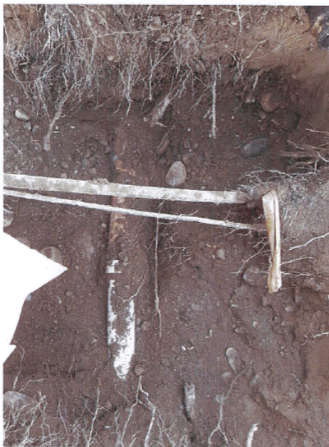
Root intrusion and repair Te Anau
