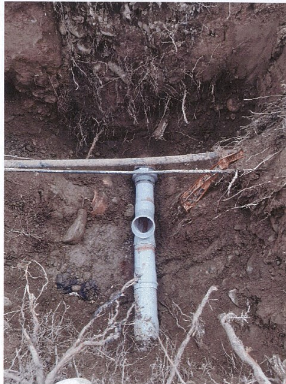
Root intrusion and repair Te Anau
