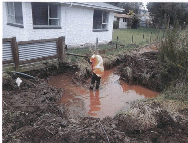
Unblocking Stormwater drain at Riverton
