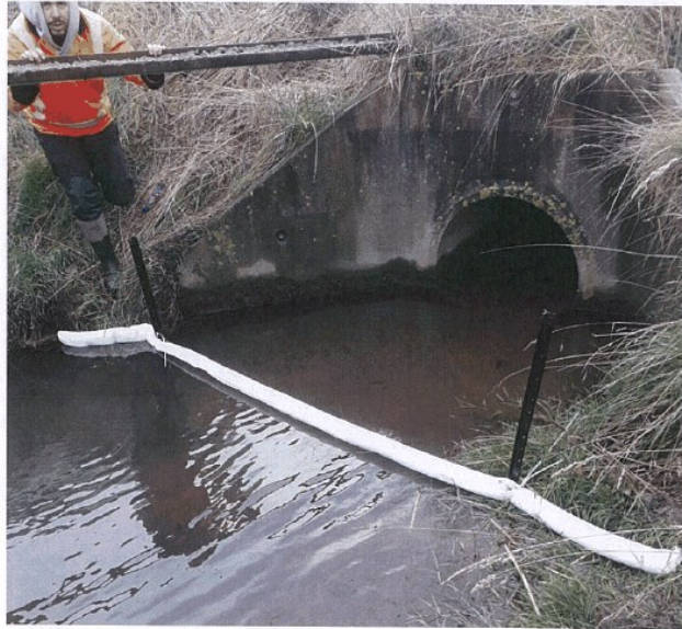
Boom installed at Winton, preventative measure
