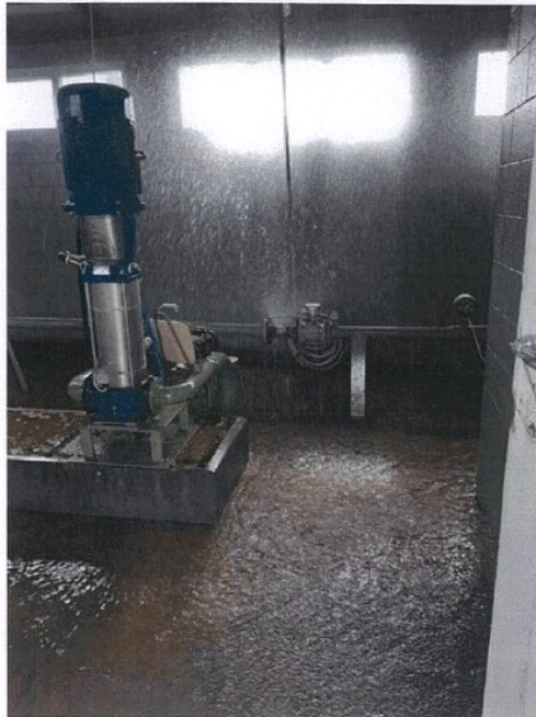
Flange gasket failure at Homestead Rural Scheme
