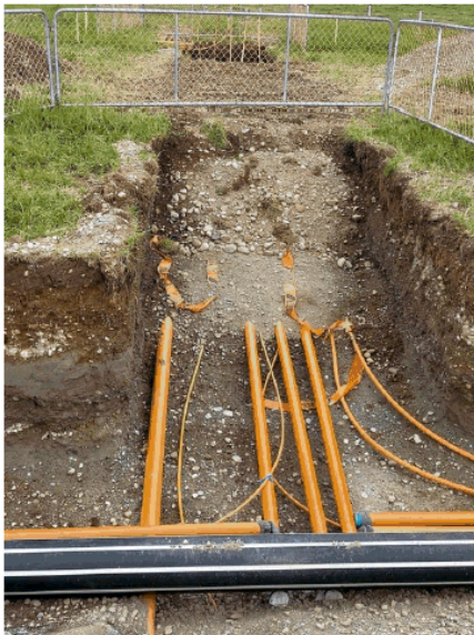
Kepler site for power conduits and fibre optic ducts, this forms a junction box of the 12 km of ducts to be installed
