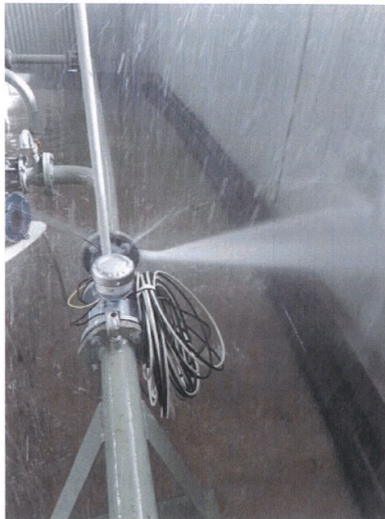
Flange gasket failure at Homestead Rural Scheme
