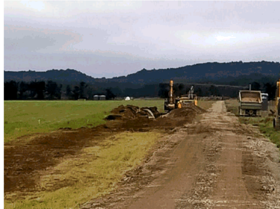
Works on site commencing with trenching laying 9 different pipes and conduits in one trench.
