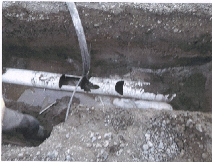
Fibre strike of 200mm rising main to the WWTP at Riverton
