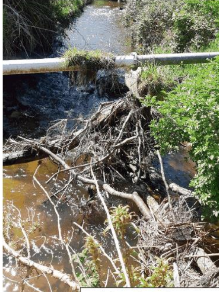
Debris and erosion at Tuatapere around sewer main
