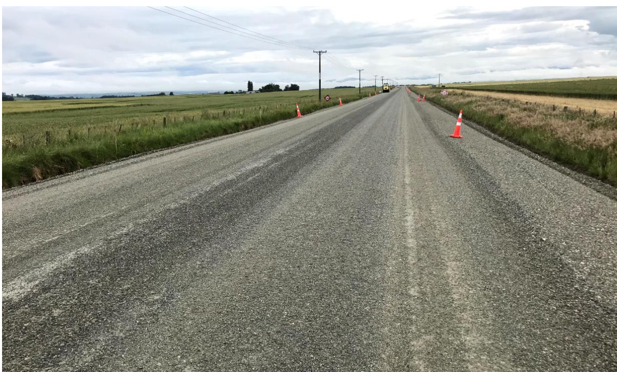
The first 1km section of Balfour Ardlussa Road rehabilitation ready for sealing
