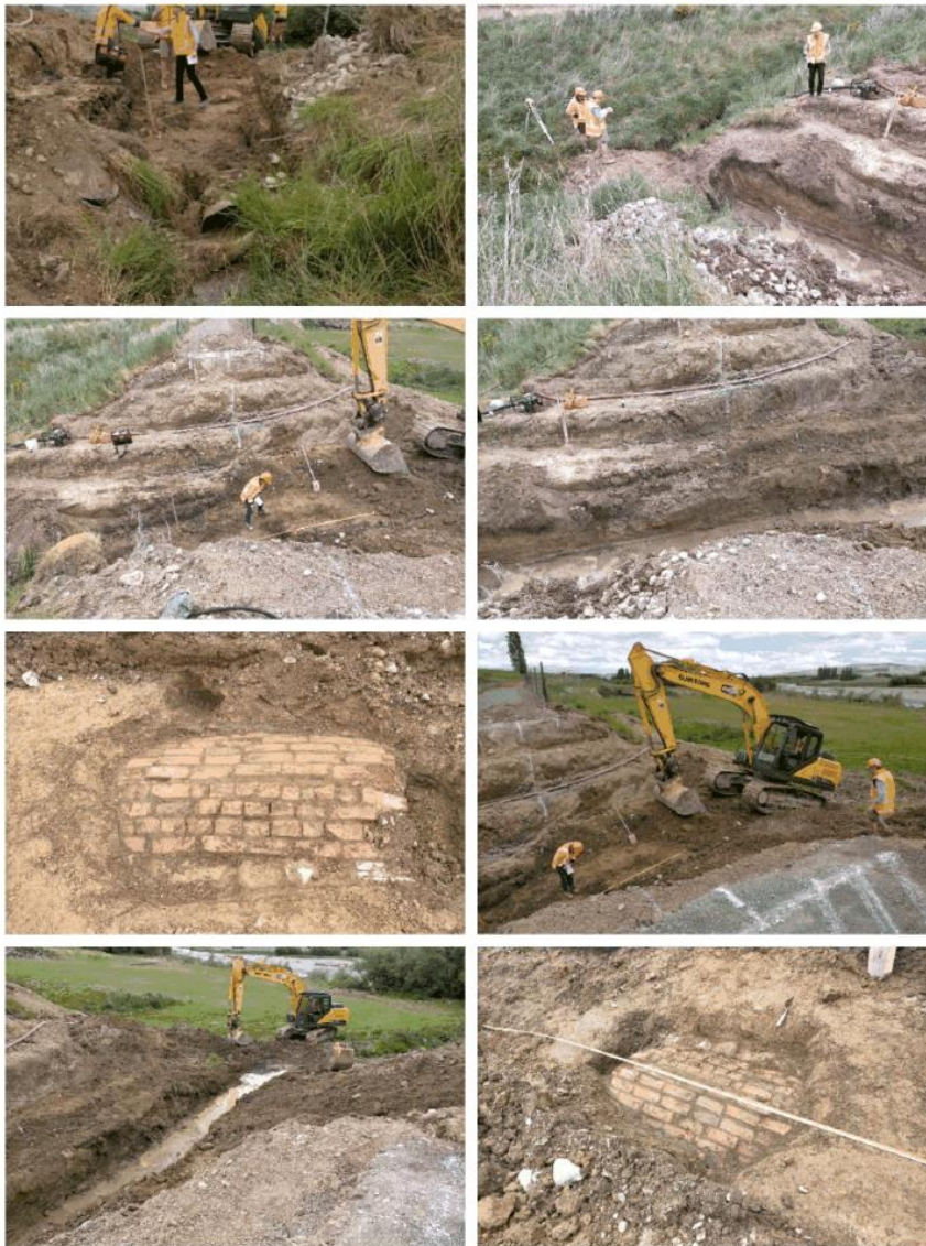
Cycle Trail culvert replacement
