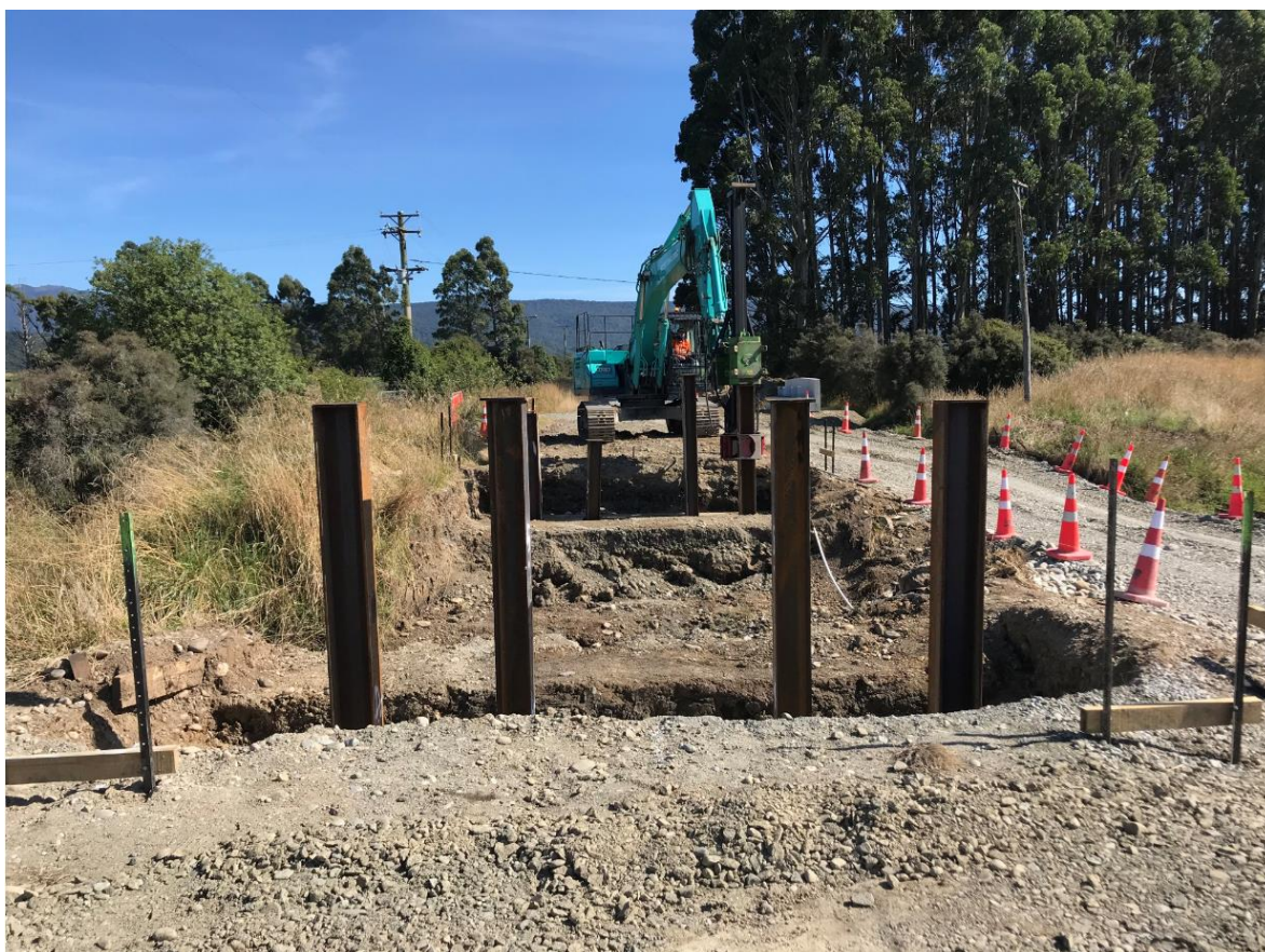
Piles being driven at Lilburn Monowai Road
