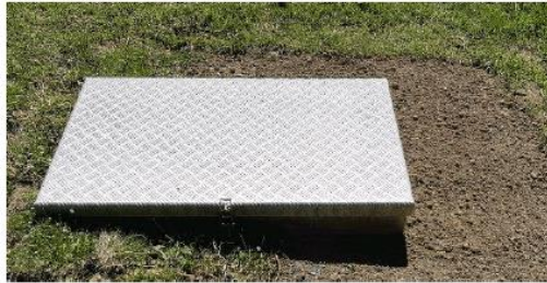
New valve pit lid installed at Stewart Island
