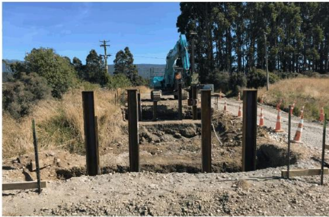
Piles driven at Lilburn Monowai Road Bridge
