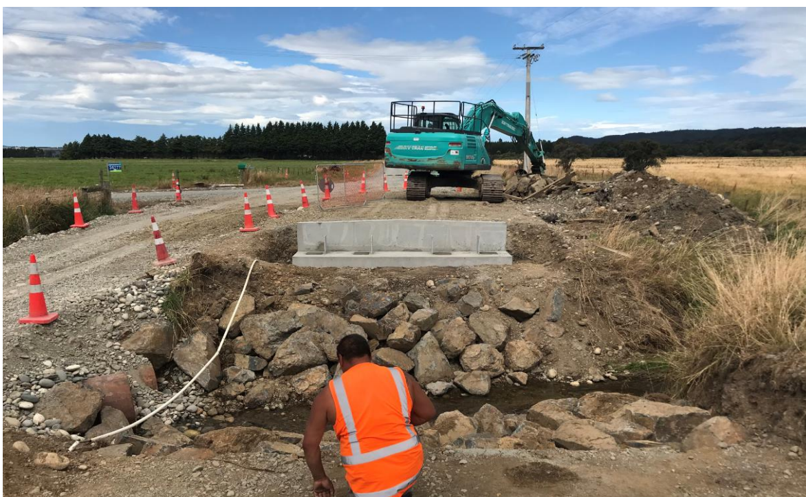
Precast abutments installed at Lilburn Monowai Road
