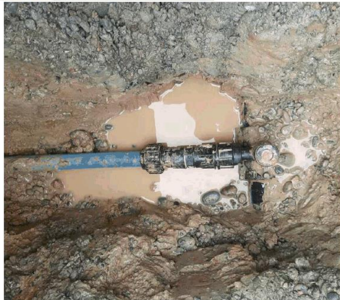
Fitting failure lateral to the main
