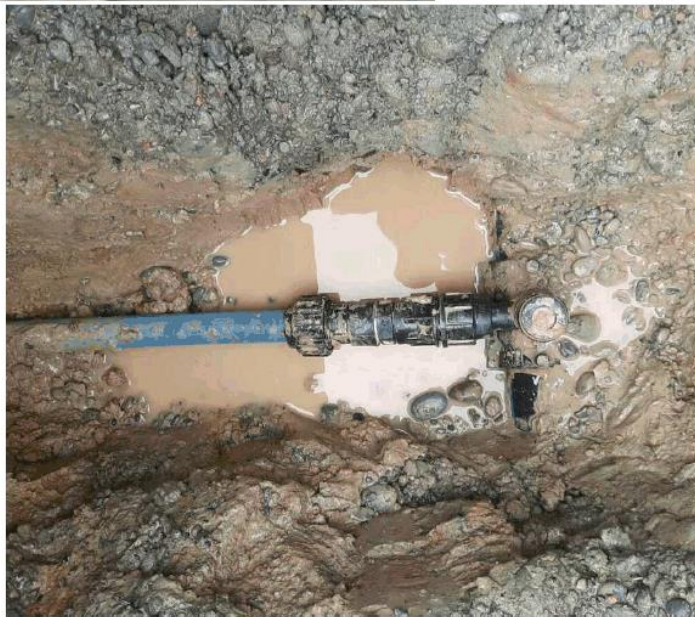
Fitting failure lateral to the main
