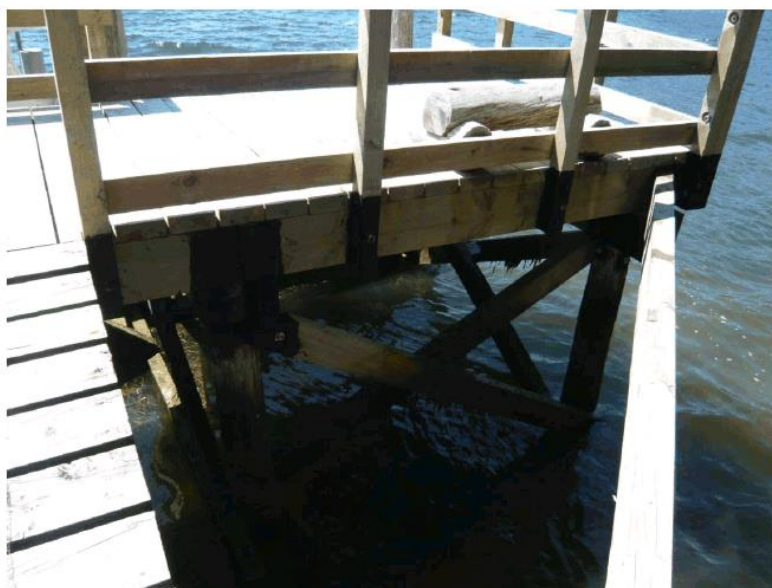
Photo 4 - FREDS CAMP - Tee-head structure and tie/brace
