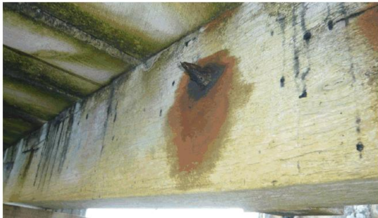
Photo 26 - ULVA ISLAND - Typical handrail connection
