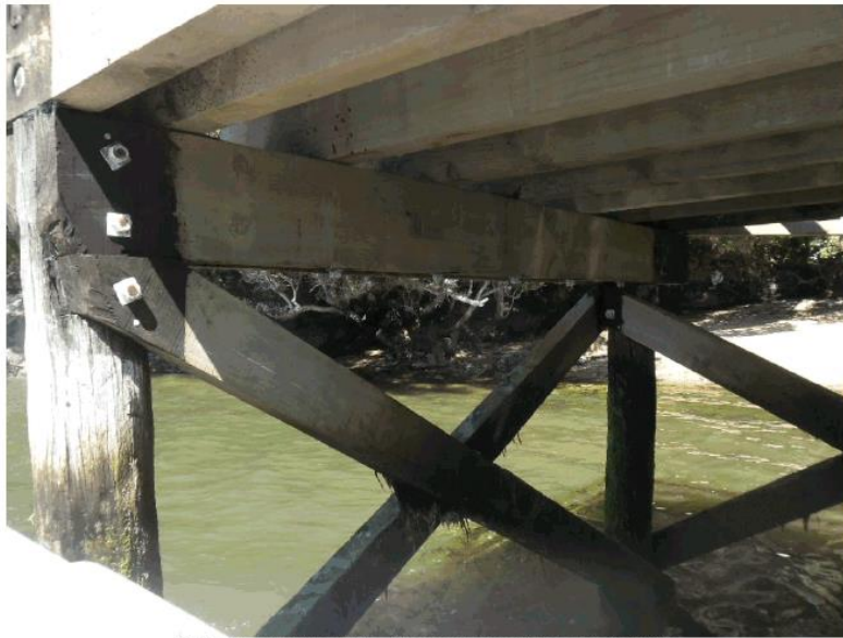
Photo 5 - FREDs CAMP - Underside of outer deck structure
