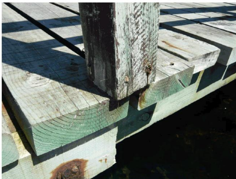
Photo 15 - MILLERS BEACH - Handrail deck fixings
