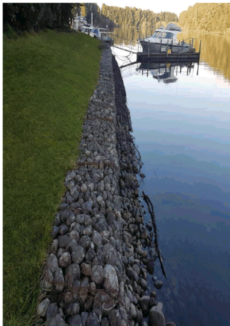
View of the deterioration of the existing Gabion basket which are stabilising the shoreline.
