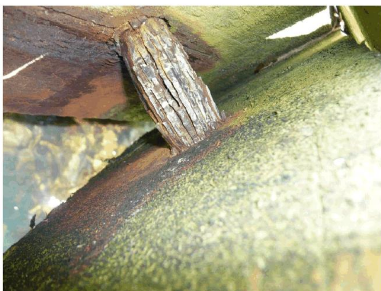
Photo 16 - MILLERS BEACH - Typical unprotected fixing
