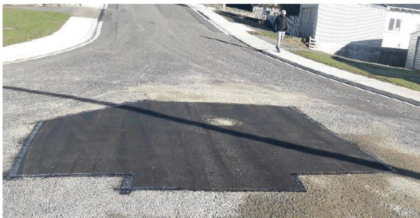
Verdun Street, Riverton – showing sewer lateral broken going through SW main and manhole installation after repair
