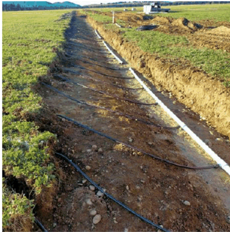
Flush side of dripper lines in fields 3 & 4
