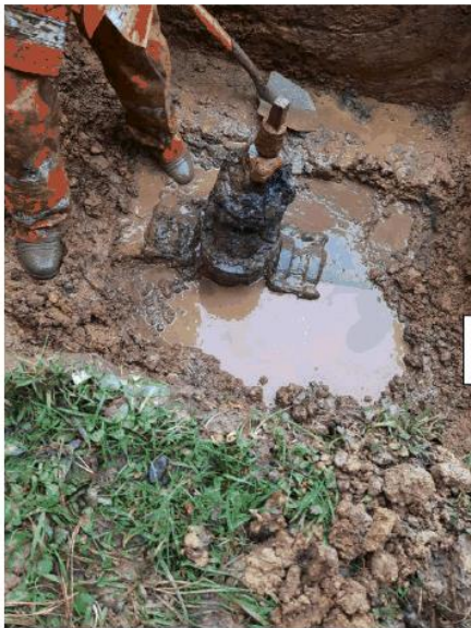
Replacing a 200mm valve in Riverton
