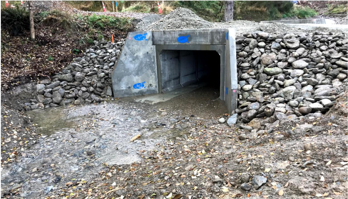
McLean Road box culvert under construction
