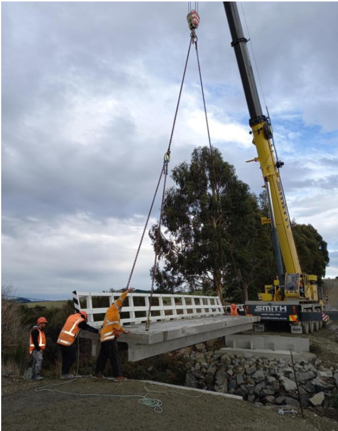
Final stages of the bridge being realigned at Biggar Road
