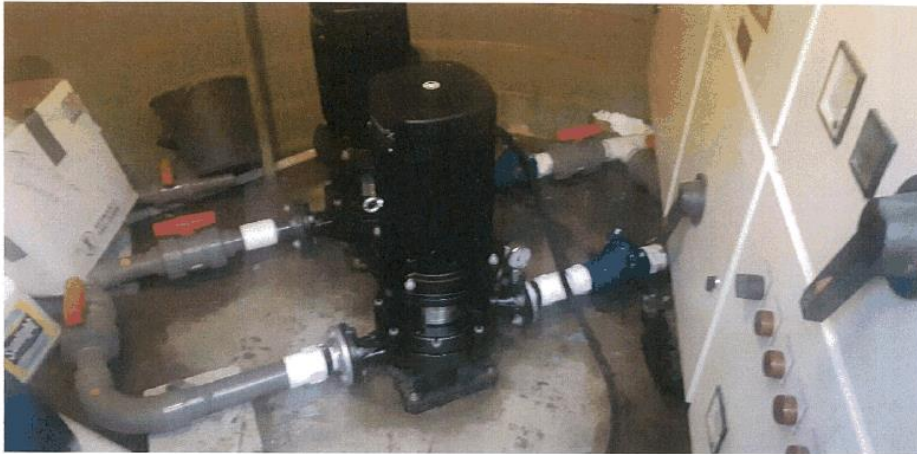
New pump installation supplying the distribution fields at Stewart Island
