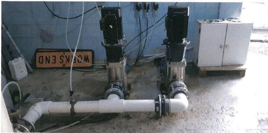
New filter pump install at Tuatapere
