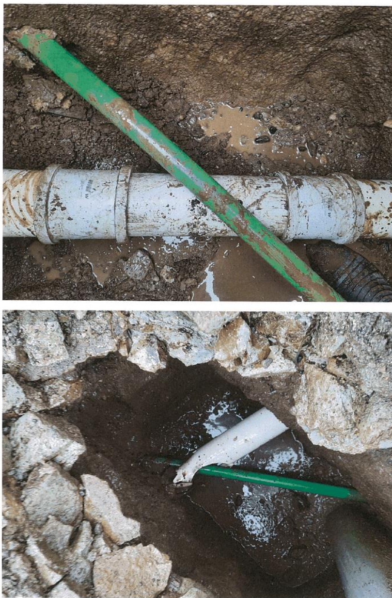
Shrewsbury Street, Riverton fibre strike
