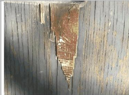
Plywood delaminating
