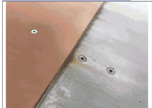
Monitor rust at top of ramp
