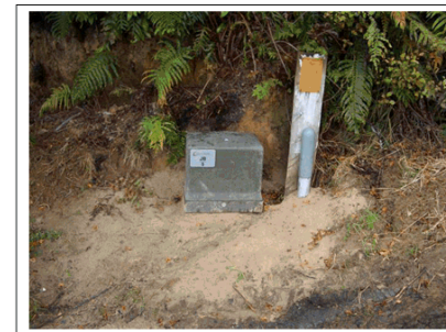
Link Box 5 (Excelsior Road) has been replaced after a motor vehicle accident earlier in the year
