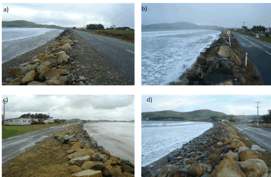
Figure 4 - Existing rock revetment along Colac Foreshore Road showing a) view west along 2012 emergency works with "rotten-rock" backfilling of road verge, b) view west at the eastern entrance to Colac Bay township with large 1 m boulders placed on road verge, c) view east from Colac Bay Road 'T intersection' with wider grass verge, and d) view west towards Bungalow Hill from near the 'Pavilion' restaurant (25 May 2015).
