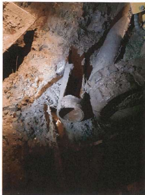
Lumsden mains failure 150 AC in very wet area
