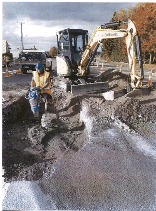
300mm valve replacement on Milford Road
