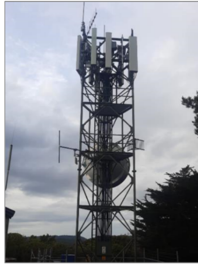
Figure 8. Oban Tower – Stewart Island RCU2.
