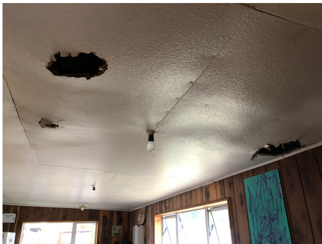
Figure 2 Water damaged ceiling in kitchen
