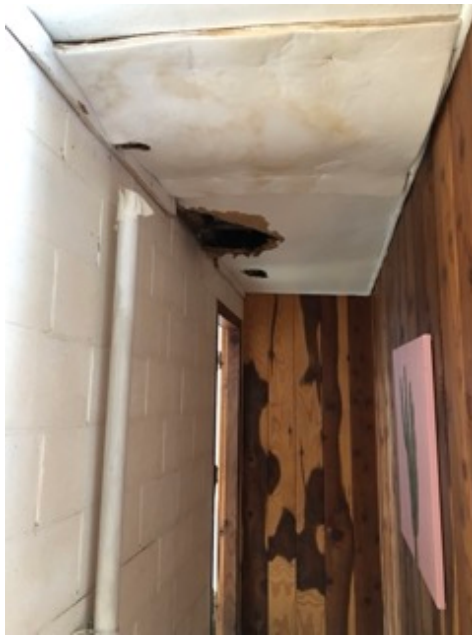
Figure 4 Water damaged ceiling in corridor
